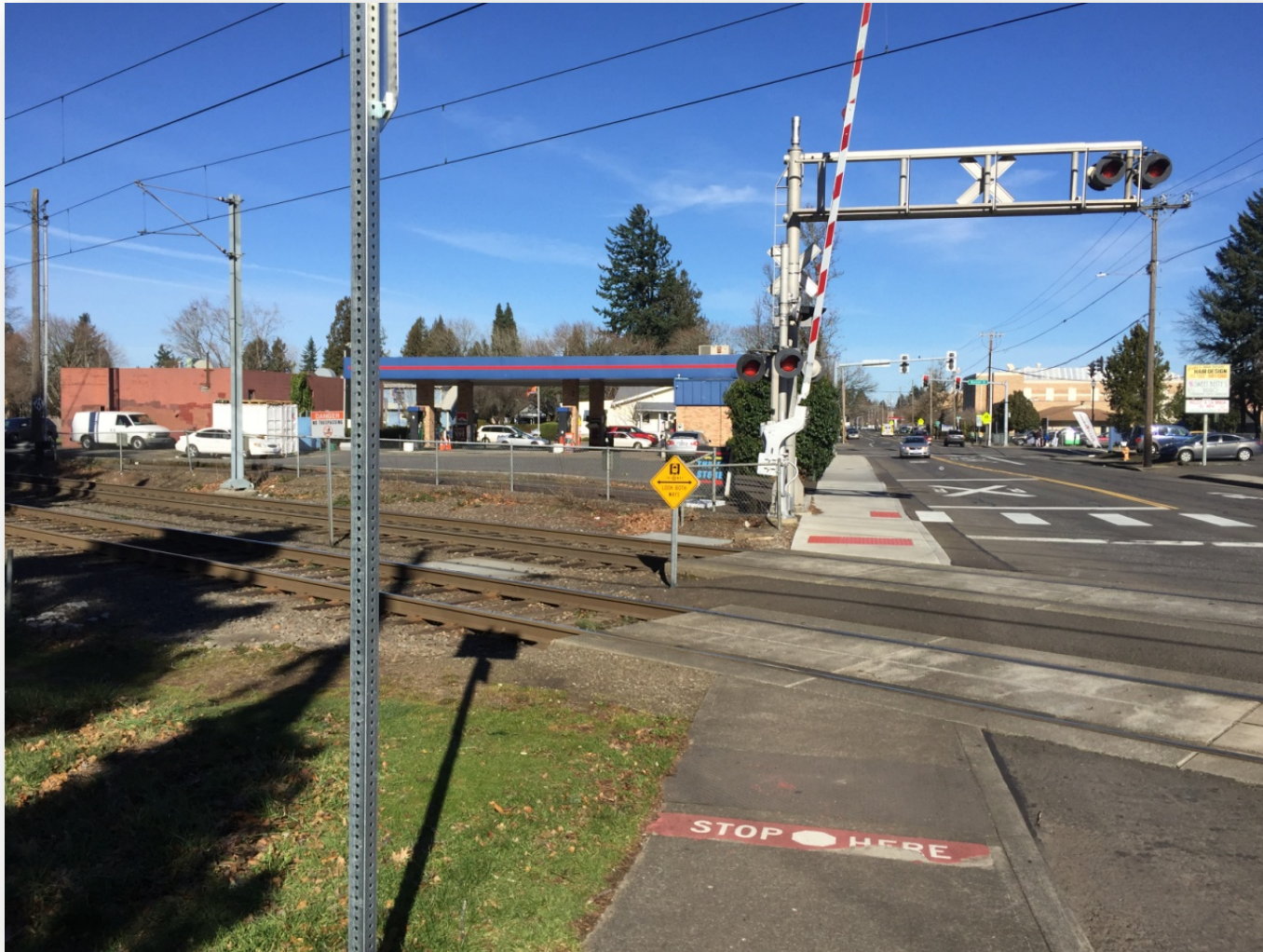
Typical existing conditions at a MAX gated crossings
