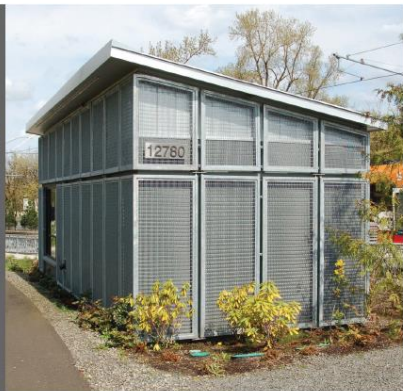
SYSTEMS BUILDING WITH METAL SCREEN IMAGE SOURCE: ZGF
