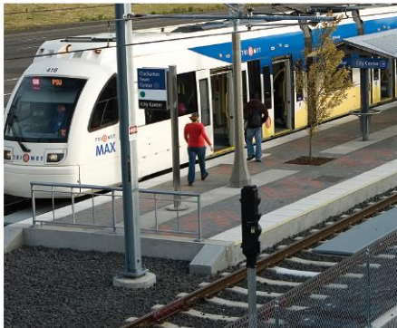
BALLASTED TRACK AT DEDICATED LIGHT RAIL STATION
