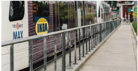
PLATFORM RAILING IMAGE SOURCE: TRIMET FLICKR
