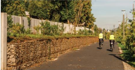
GABION WALL IMAGE SOURCE: MAYER/REED
