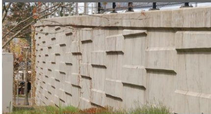
WALL WITH PATTERN RELIEF IMAGE SOURCE: ZGF
