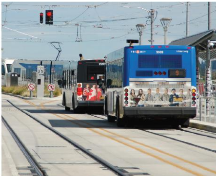
EMBEDDED TRACK ON SHARED TRANSITWAY
