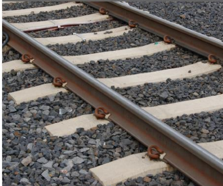
BALLASTED TRACK DETAIL
