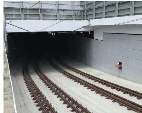
DIRECT FIXATION TRACK THROUGH TUNNEL
