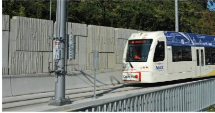
LARGE PANEL TEXTURED WALL IMAGE SOURCE: PETER EHRLICH
