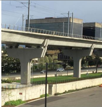
TYPICAL CONCRETE COLUMNS AND GUIDEWAY STRUCTURE
